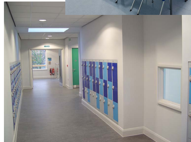
First floor Corridor & Lockers
