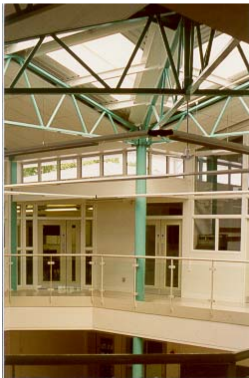
Ventilation Tower and Daylighting
