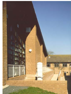
Entrance / Link to New Building
